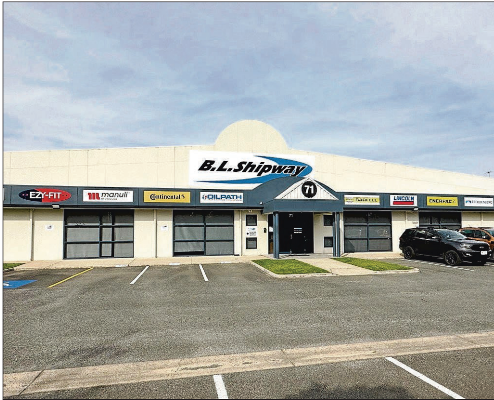
David, Todd and the whole Shipways team look forward to continuing to service past, present and new customers in an even better way from their new expanded premises at 71 Morphett Road, Camden Park. Picture supplied
